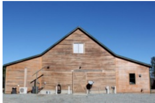
Rear of Custom Barn
