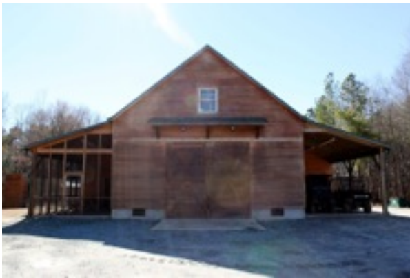
Front of Custom Barn
