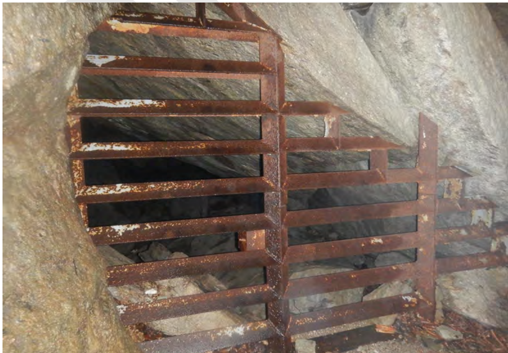
FIGURE 11. Installing gates or fences at hibernaculum sites threatened by human activities is one conservation action biologists can do to protect VBEB habitat.
