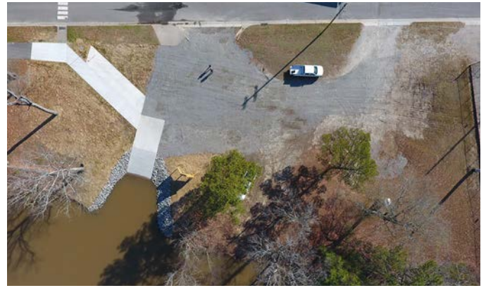
Overhead view of Sunset Park Boating Access Area in Rocky Mount. This project won a States Organization for Boating Access award in 2021. It was designed by division Engineer Michael Leggett; built by the Rhodes Pond construction crew.
