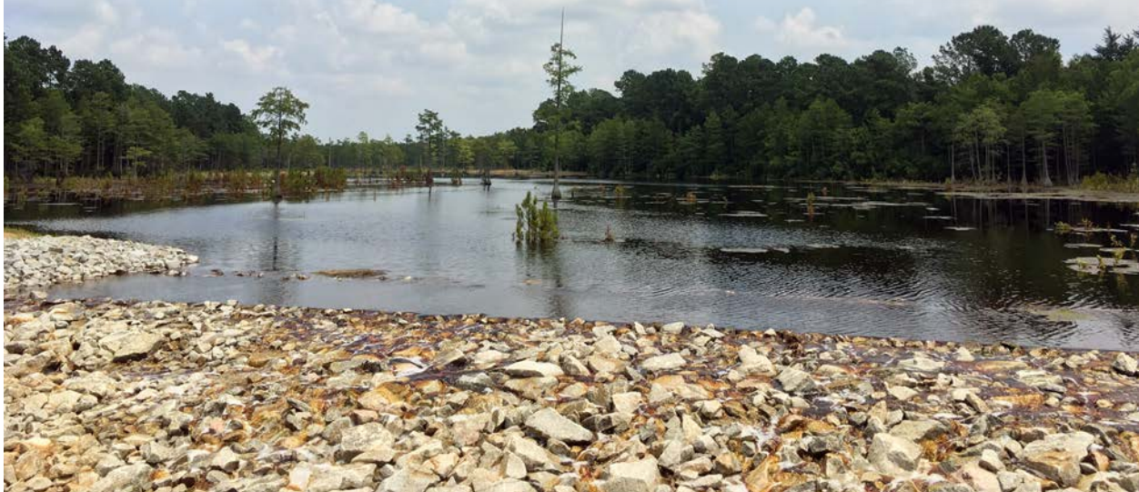
Restored Jessups Mill Pond, in Cumberland County, following the dam reconstruction project.
