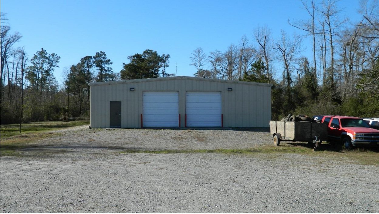
Front View of 50x50 Building - Tract B
