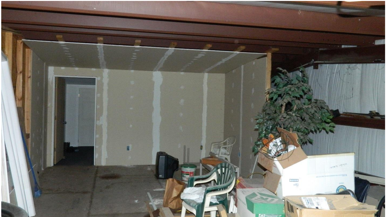
Overhead Storage Area – Tract A
