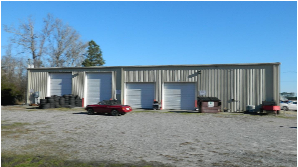
Rear View of Building – Tract A
