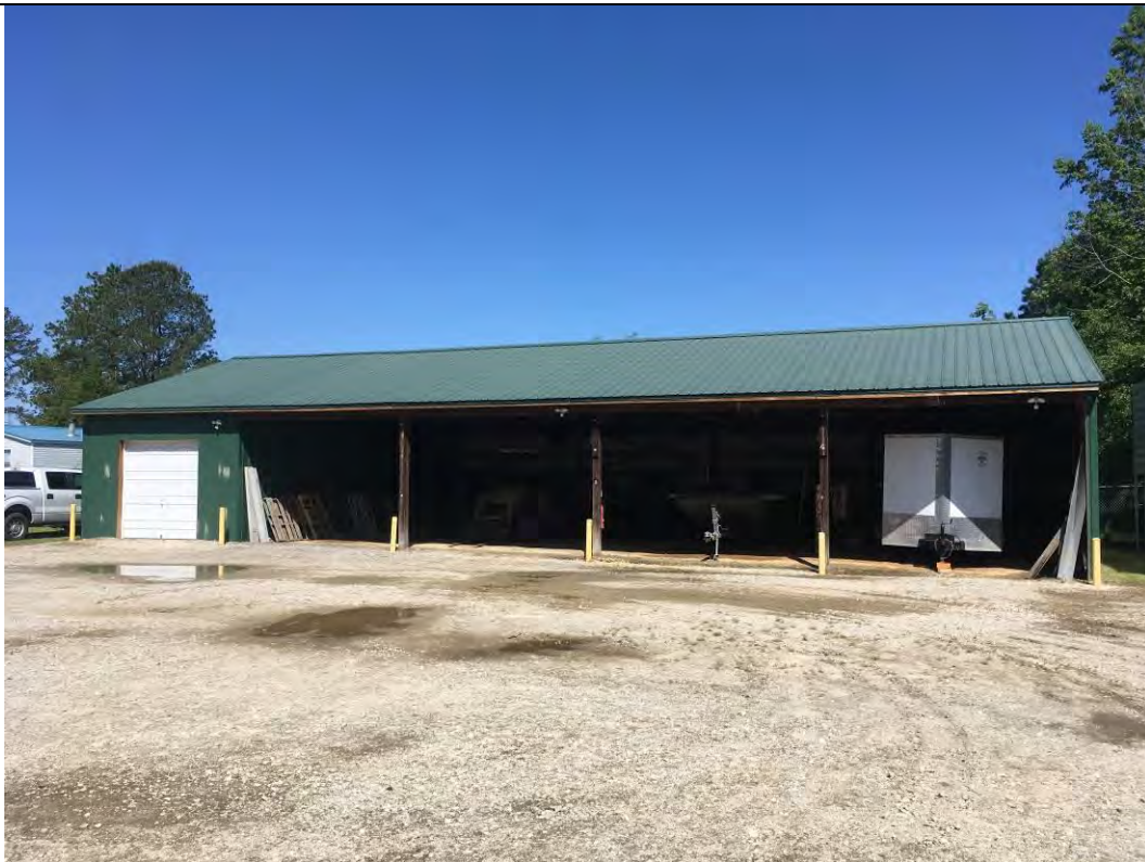
Photo 1: Front of Elizabethtown Pole Shed
