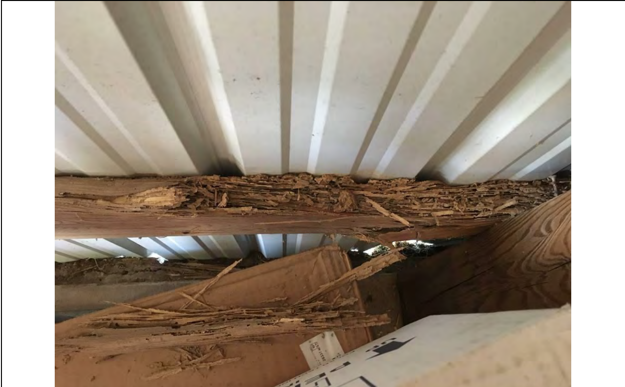
Photo 2: Severe termite damage of timber girt that provides bracing and attachment point for siding
