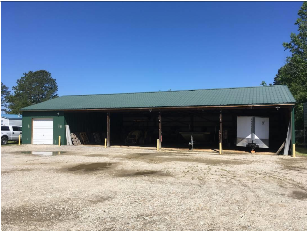
Photo 1: Front of Elizabethtown Pole Shed
