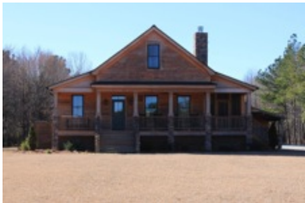
Front View of Lodge
