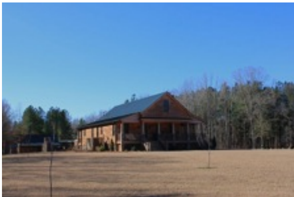
Corner View of Lodge
