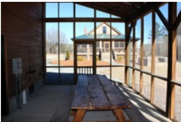
Screened in Porch on Barn
