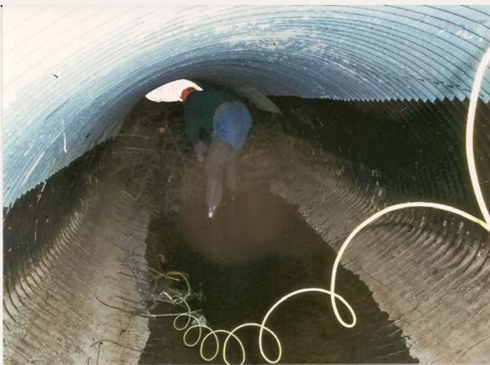
Above: Wildlife specialist rigging a delayed explosives detonator to remove a beaver dam clogging a DOT pipe in Nash County.
