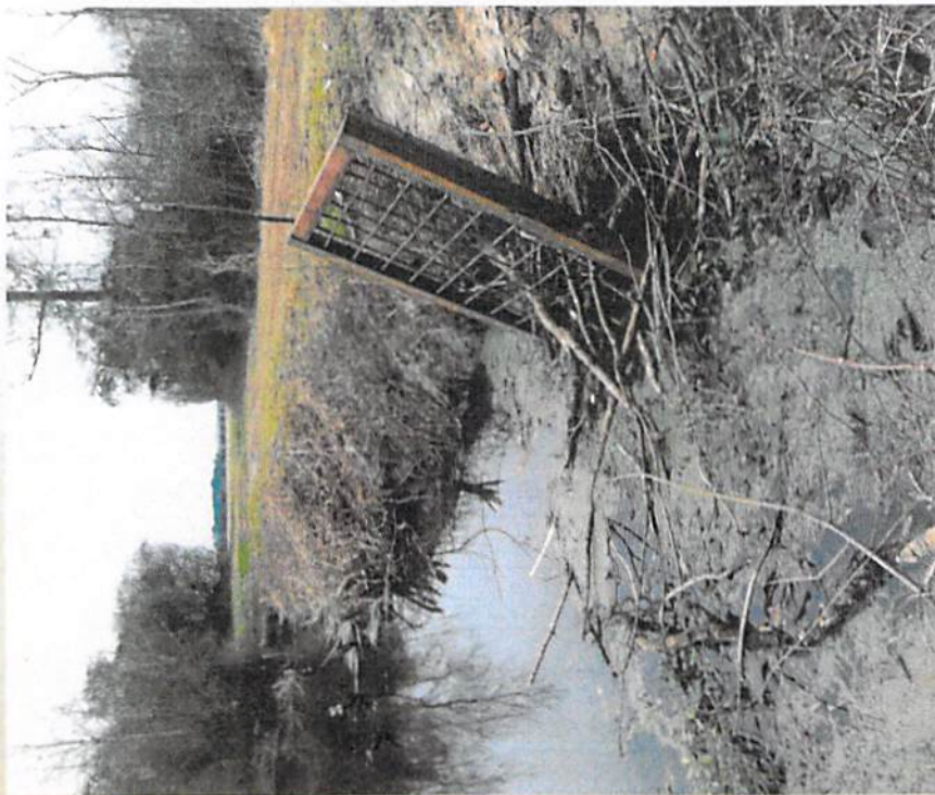
Pond bank damaged after beaver plugged an overflow pipe in Pender County.
