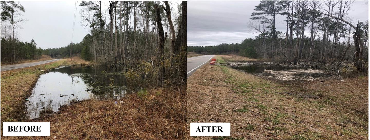
The photos above are from Camp Leach Road in Beaufort County where beaver dams blocked two, 48-inch culverts. Beaver damage management activities conducted through BMAP restored normal water drainage, preventing damage to the roadway and saving nearby timber from flood damage.
