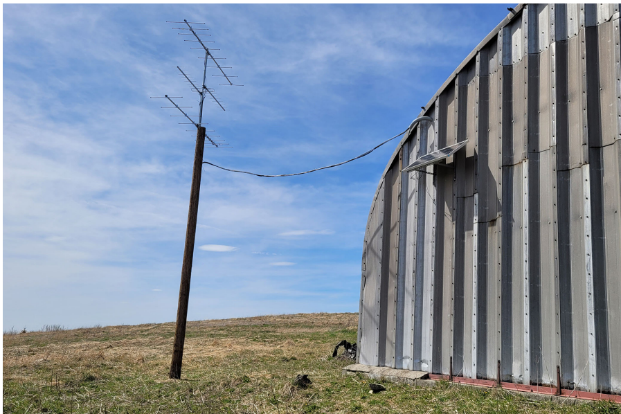
Antennas are mounted on the wood pole and the receiver station is housed inside the hangar, safe from the elements (Chris Kelly).
