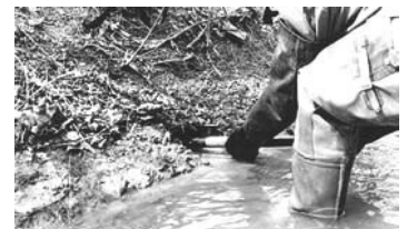
Dig pocket at water line
